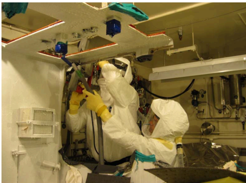
Worker using HEPA filtered vacuum to clean a beryllium area. Image source: beryllium practitioners guide 2nd edition
